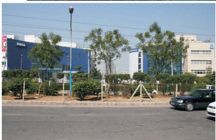
Vipul TechSquare, Gurgaon
