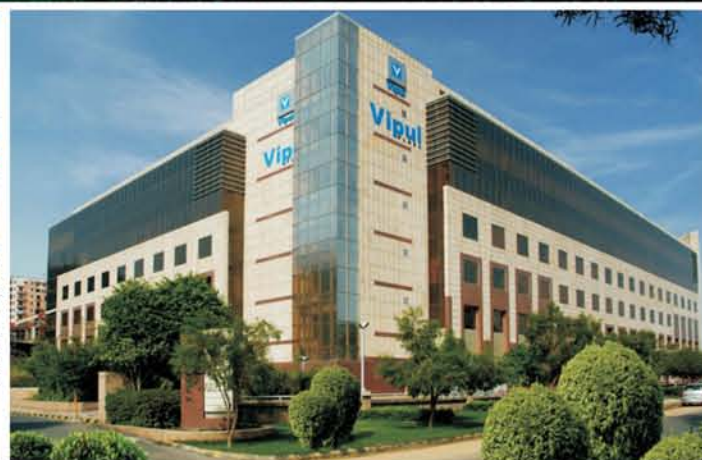
Vipul Plaza, Gurgaon
