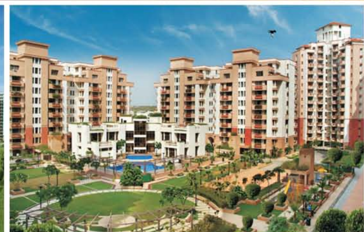
Vipul Gardens, Gurgaon
