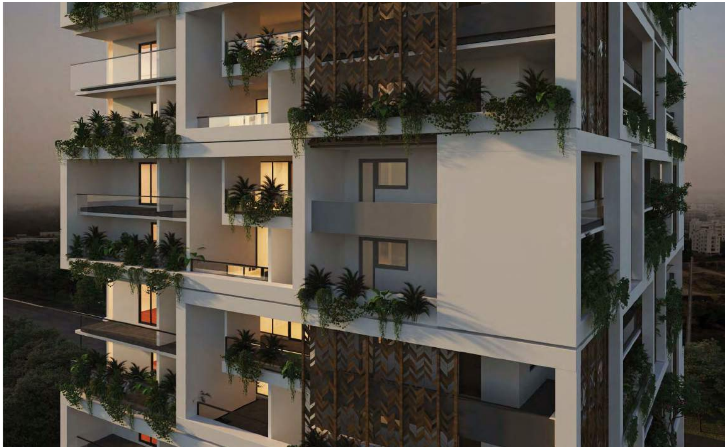
Rear view building facade
